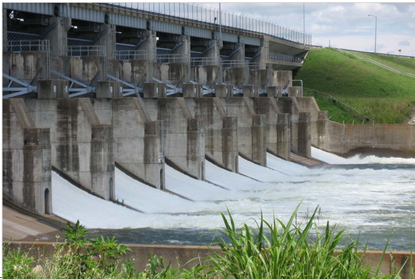
First Day Water Released at Lake Lavon Dam
